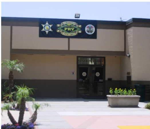
Los Angeles County Sheriff's Department Substation in the City of Pico Rivera . Ronald Bates is the Pico Rivera City Manager.
