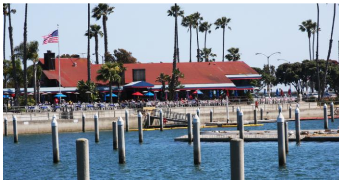
Boat slip improvement project underway in Long Beach .
