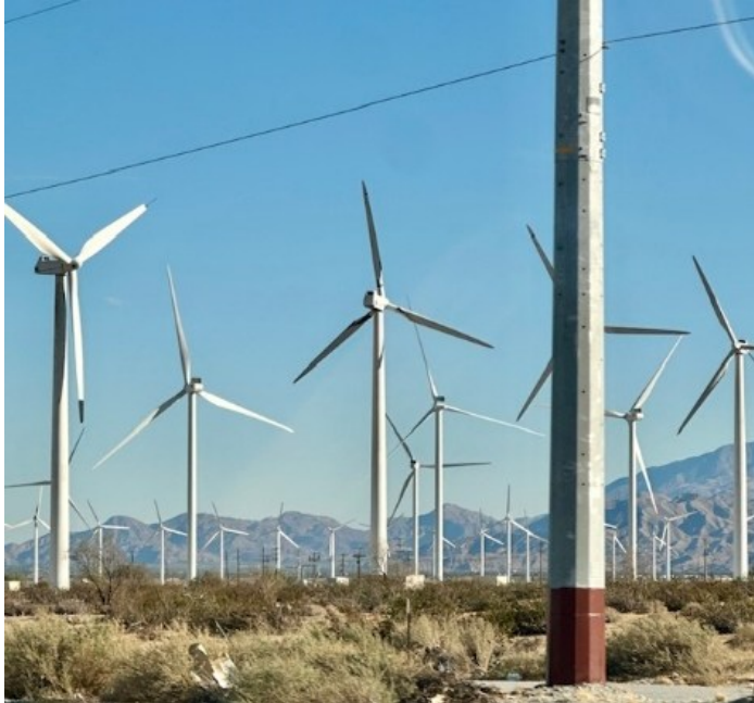
Windmills in the Coachella Valley generate enough electricity to power the entire region, including Palm Springs . Development of the windmill farm began in the 1980s. It is one of the first three such farms in California, along with Altamont and Tehachapi passes.
