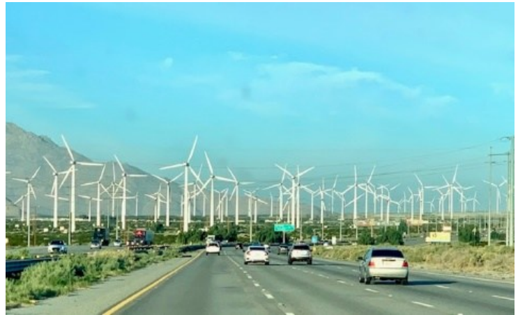
Windmill production of electric energy.
