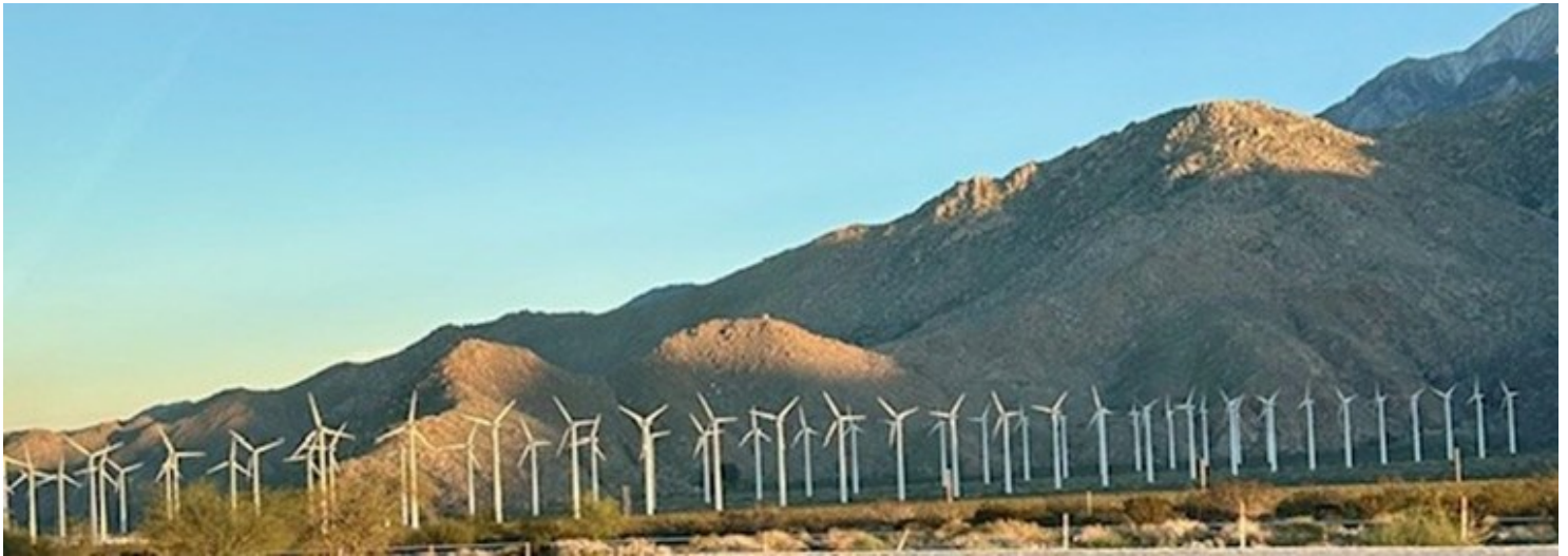
Part of the San Geronio Pass wind farm in the Coachella Valley. It features more than 650 active turbines that produce a total capacity for about 656 megawatts. Enough electricity to power the entire Coachella Valley; 10% of the State of California's wind energy.
